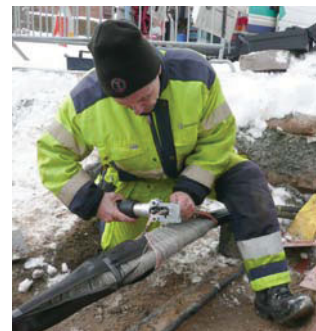
Crimping with Elpress crimp tool PVL611.
