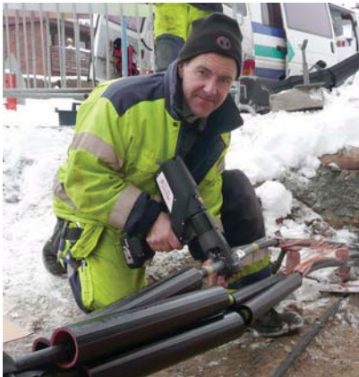
Crimping with Elpress crimp tool PVL1300.
